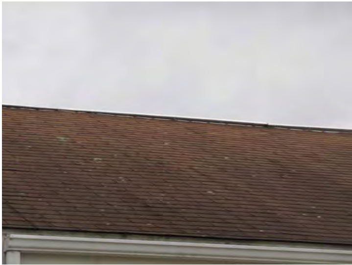
Original three-tab shingles on roof of Building #316
