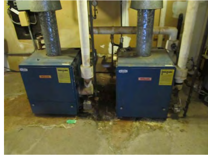
Typical original boiler plant at each residential building for production of hydronic heat
