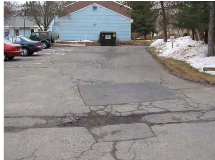
Asphalt paving exhibits age-related wear and deterioration
