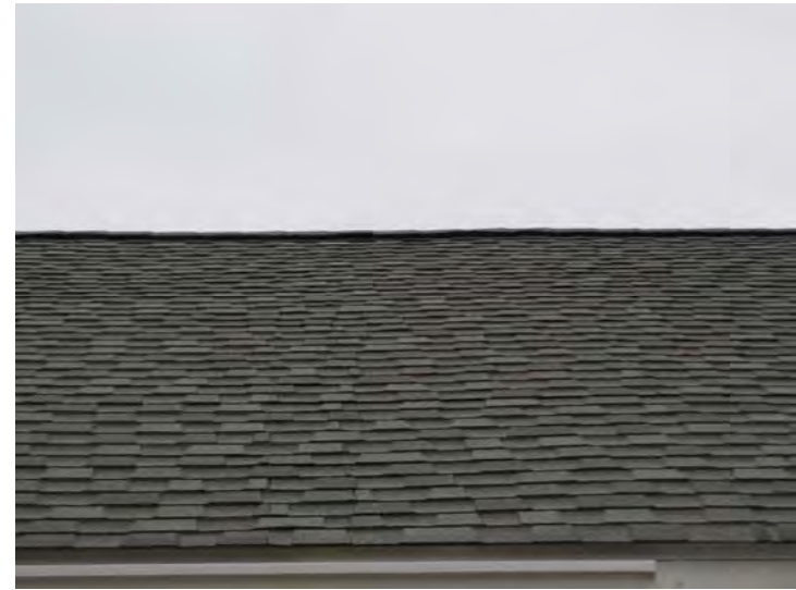
Newer architectural-style shingles typical on roof surfaces of all other buildings
