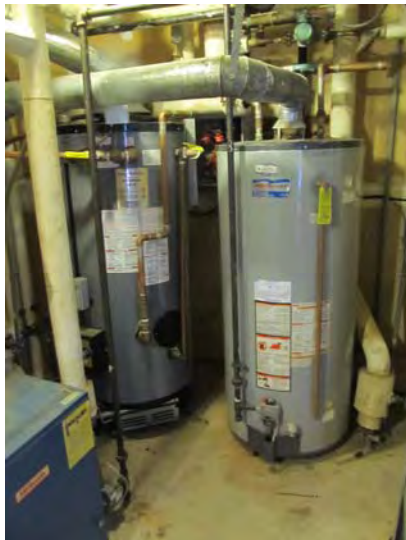
Typical freestanding tanks for production of domestic hot water at each residential building
