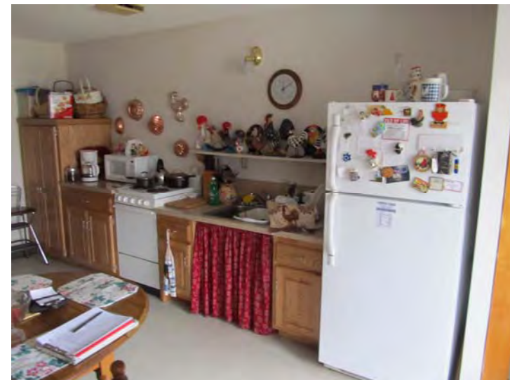
Handicap accessible unit kitchens include knee clearance space under the sink but lack a thirty-inch wide work surface with knee clearance space
